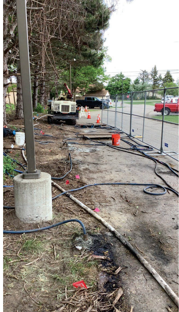
Photo G.8 Inside Work Area Fence – East End
