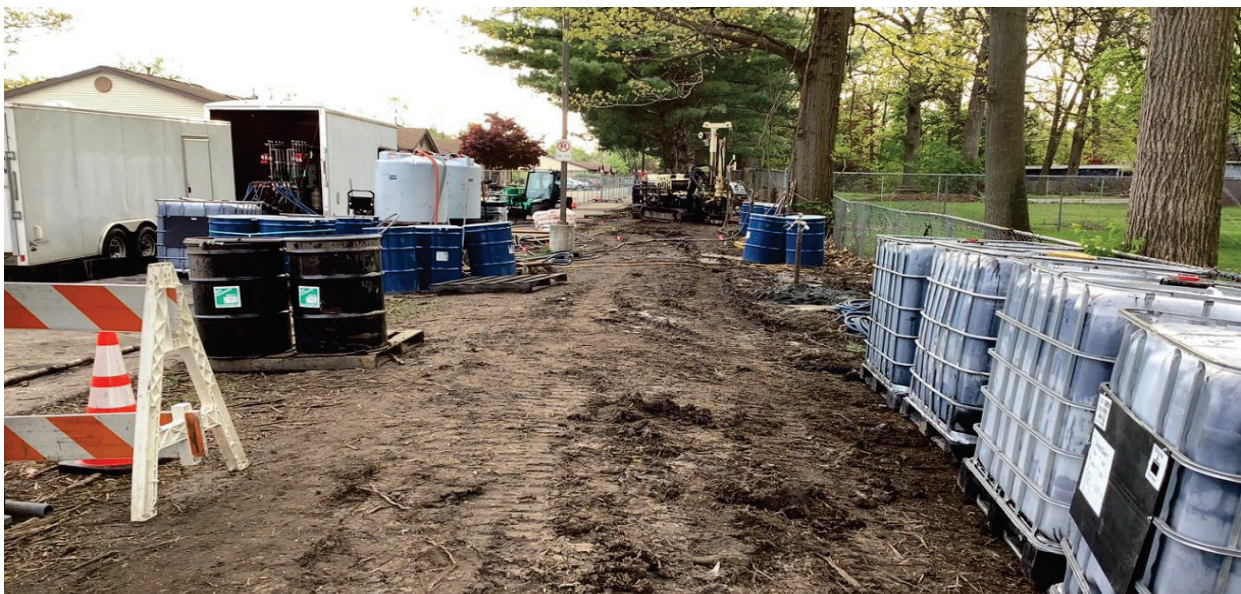
Photo G.9 Inside Work Area – Center of Work Area
