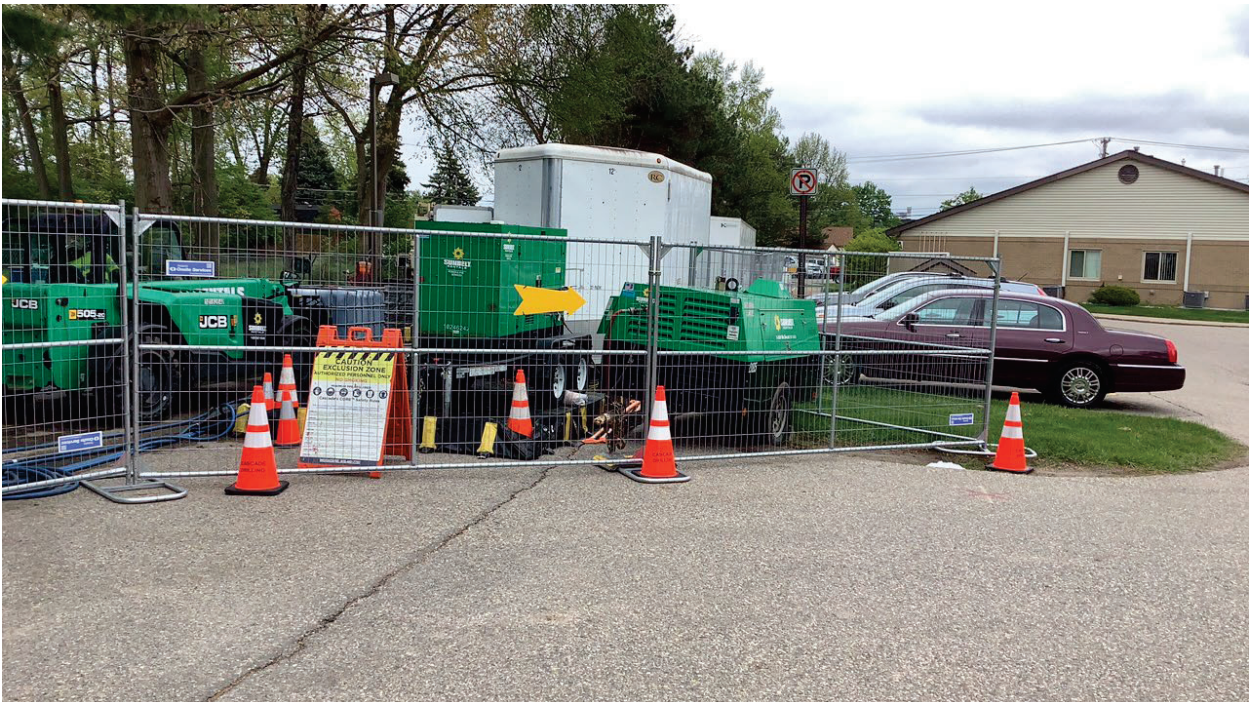
Photo G.6 Work Area Safety Barricade
