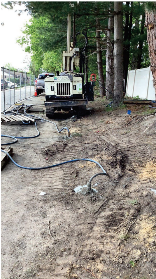
Photo G.11 South Row Injection Points and Geoprobe advancing an injection point
