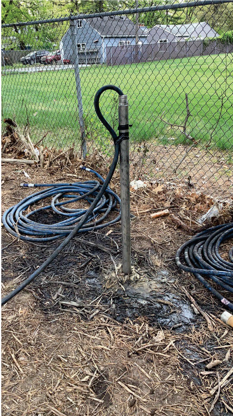
Photo G.15 Example of Shallow Interval Daylighting – N24
