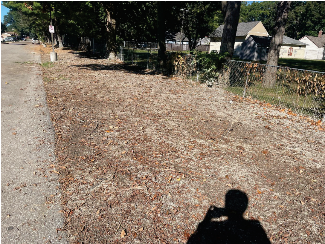
Photo G.17 Restoration - Looking West
