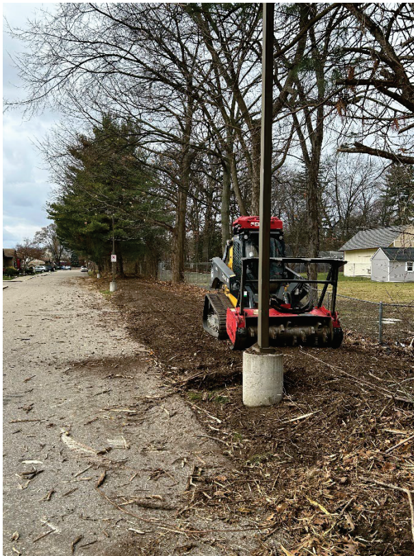
Photo G.4 Brush Clearing
