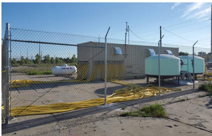
Plant 2 Biosparge Unit and Nutrient Injection Tanks
