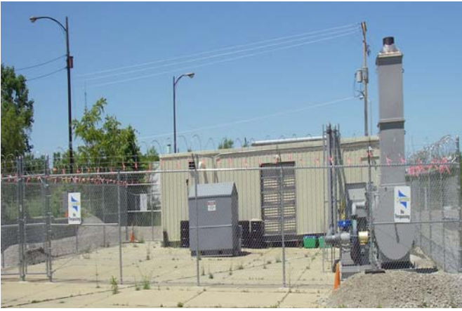
This building contains a treatment system that extracted/removed and treated gasoline-contaminated liquid and vapor from beneath the property.
