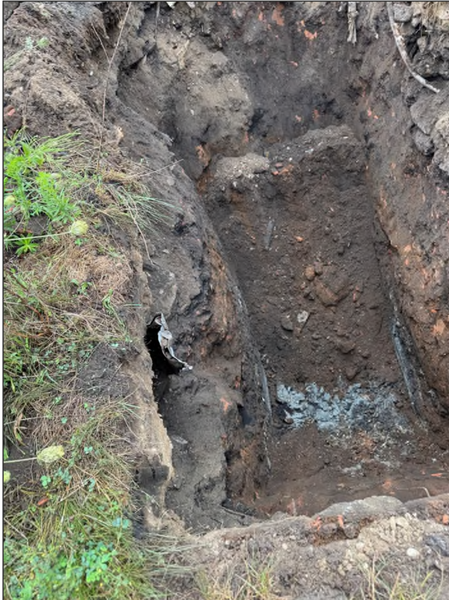
PHOTO NO. 11: Test Pit TP-10 general soil conditions.
