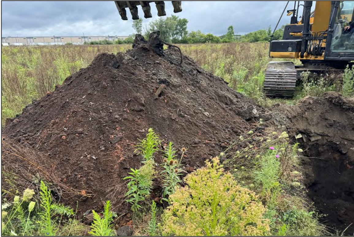
PHOTO NO. 12: Test Pit TP-10 excavated spoils.
