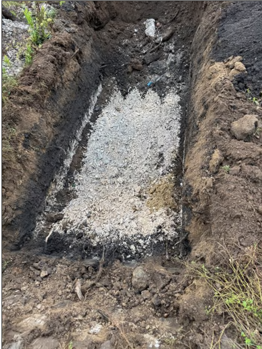
PHOTO NO. 1: Test pit TP-5 with fill soils and spark plugs.
