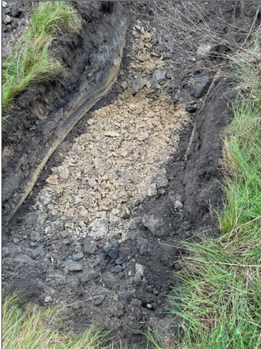
PHOTO NO. 10: Test Pit TP-9 general soil conditions.
