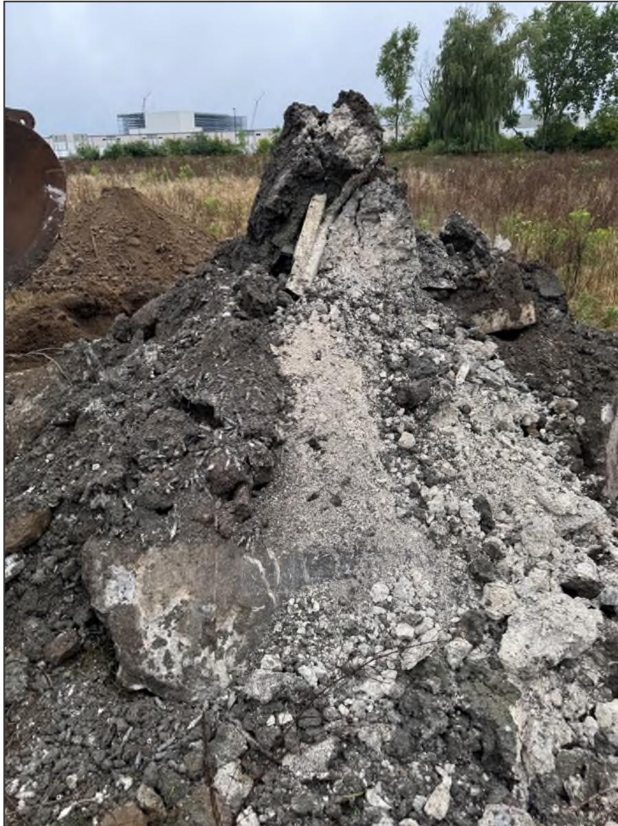
PHOTO NO. 5: Test Pit TP-6 excavated spoils.
