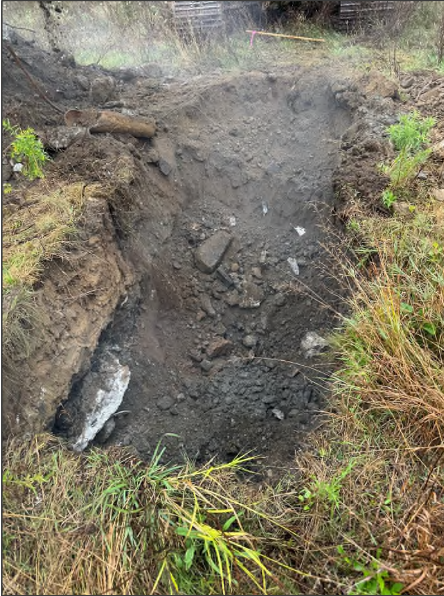
PHOTO NO. 3: Test Pit TP-6 partially excavated with concrete debris.
