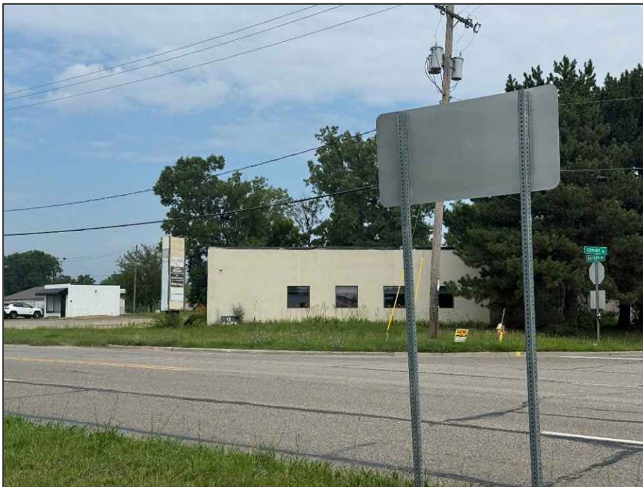
PHOTO NO. 14: View of the north-adjointing multi-tenant commercial building.
