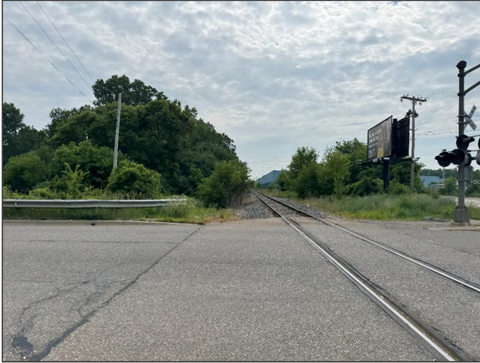
PHOTO NO. 17: View of the south-adjointing railroad line.
