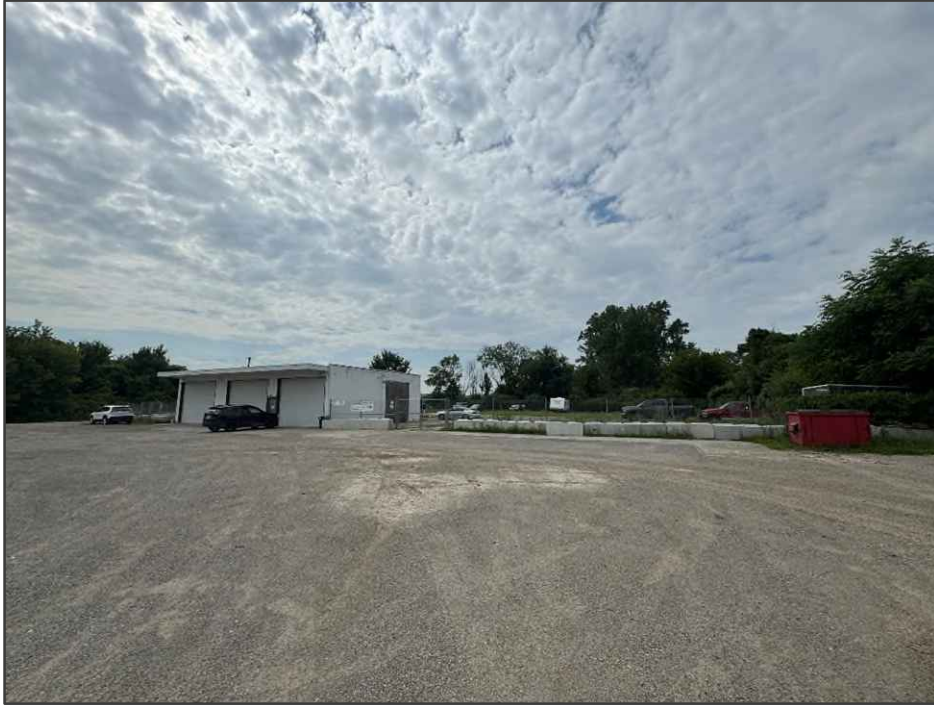
PHOTO NO. 15: View of the east-adjointing commercial building.
