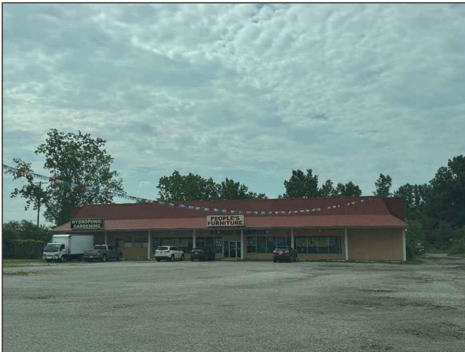
PHOTO NO. 12: View of the north-adjointing furniture store, People's Furniture, 4204 Davison Road.
