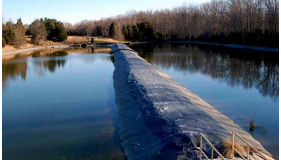
A view of detention ponds on the Property, looking south.
