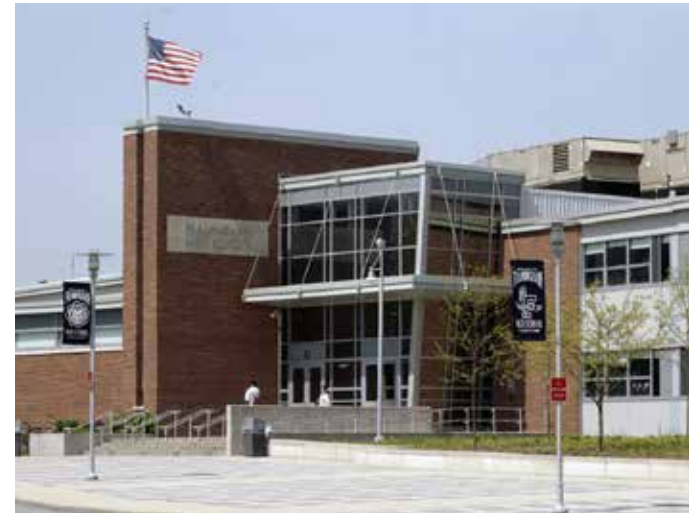
Framingham High School
